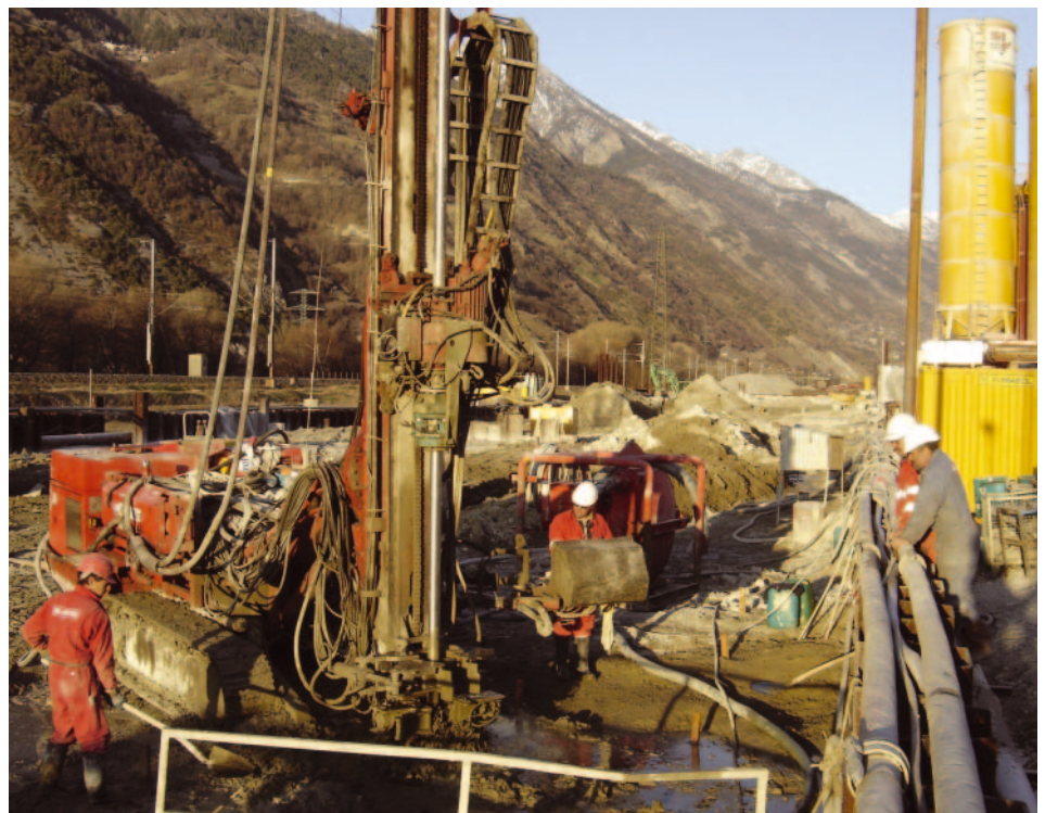
Installation de jet grouting
