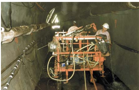
Phase de perforation
